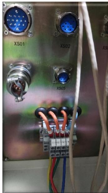
**Figure 5- three- phase input terminal**
